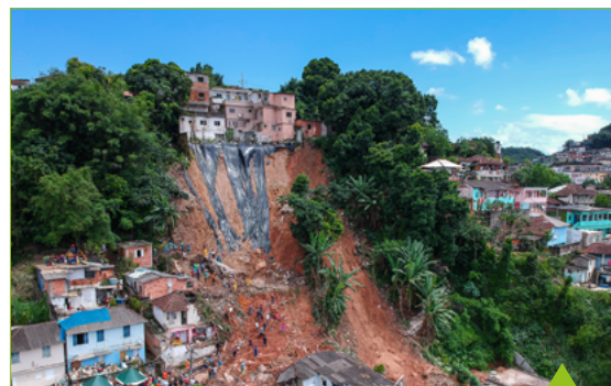
Landslide in Santos city, Brazil.
